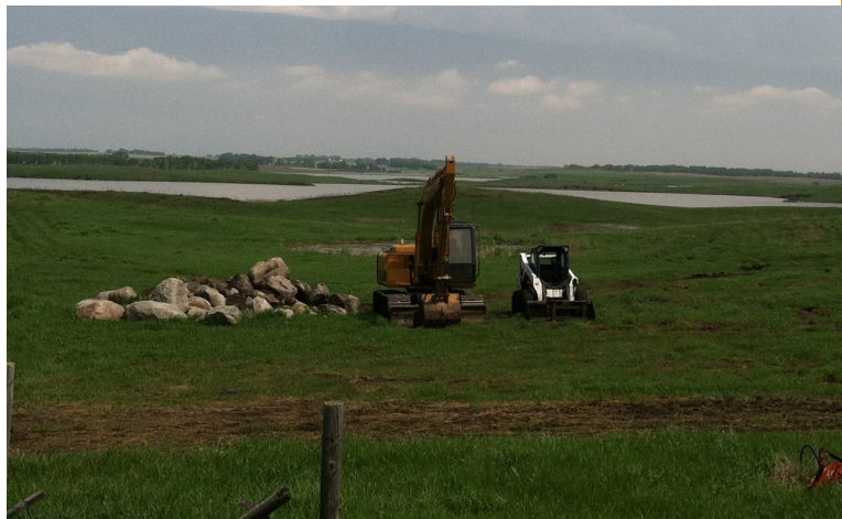
Rock clearing in preparation for prairie conversion to cropland near Clear Lake, SD (Photo by P. Bauman, 2019).
